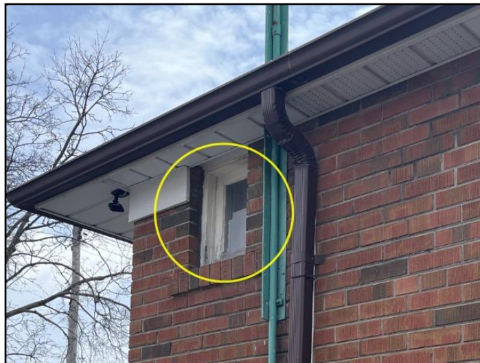
Paint and caulking - deteriorated / missing
