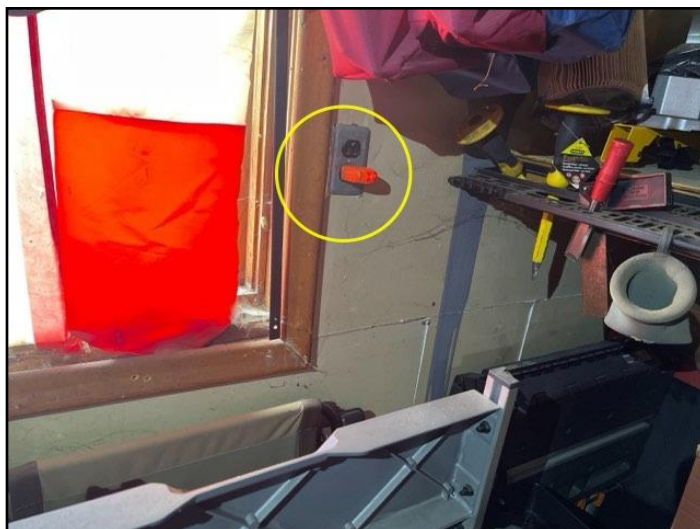
Reversed polarity
