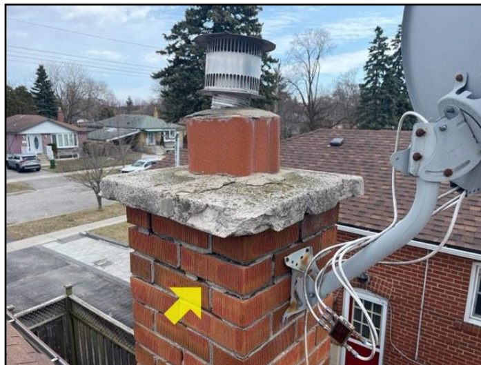
Loose, missing or deteriorated mortar
